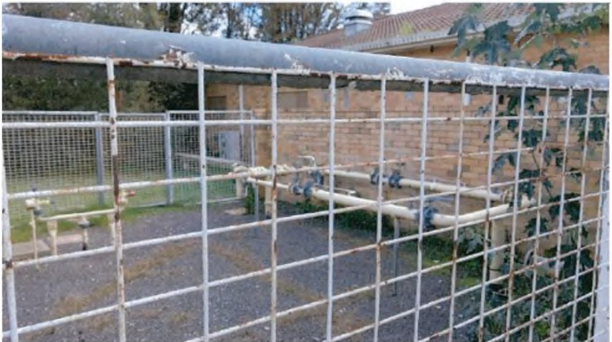
Figure G3–4: Redundant Gas Infrastructure
